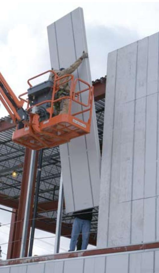
result, the ACCEL-E panels offer tested insulating values that far surpass traditional framing, sheathing and batt wall assemblies. For its recycled content, minimized waste, and energy performance, ACCEL-E contributes points to as many as four LEED categories – a fact that greatly influenced the HRDC board's decision.
