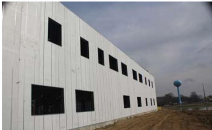
The ACCEL-E wall system combines framing and insulation to one step. The panels combine the strength of cold-formed steel framing with the insulation properties of EPS.
