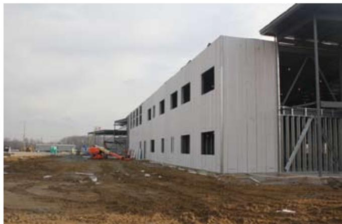
Combs Interior Specialties installed 18,500 square feet of ACCEL-E panels, approximately 80 panels.
