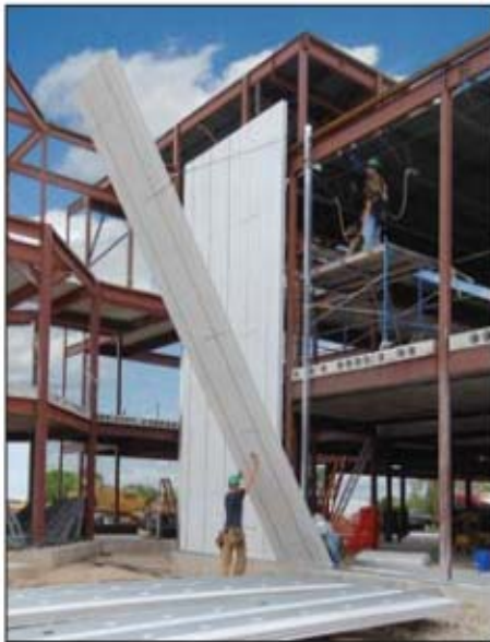
ACCEL-E wall panels can reduce labor costs and speed up construction time.
